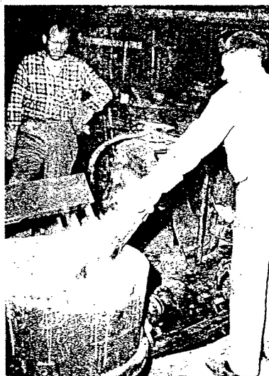
A green sapling mixes the molten metals.
