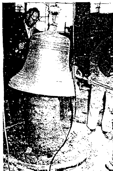
The cast bell is lifted off the core.
